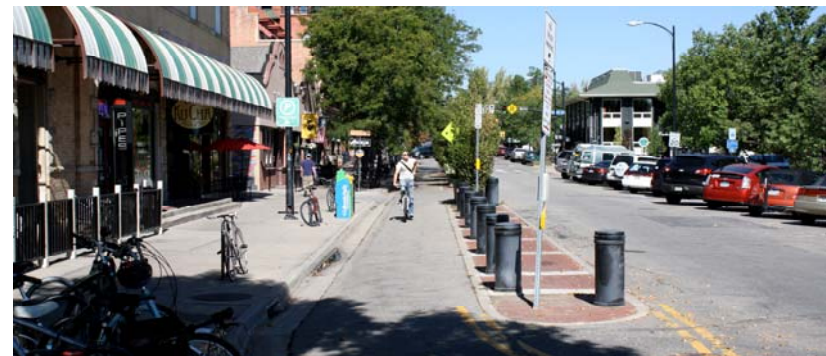
Typical separated bikeway with bollards
