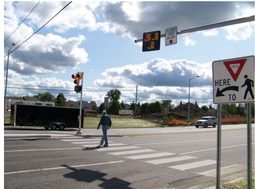
A typical pedestrian hybrid beacon
