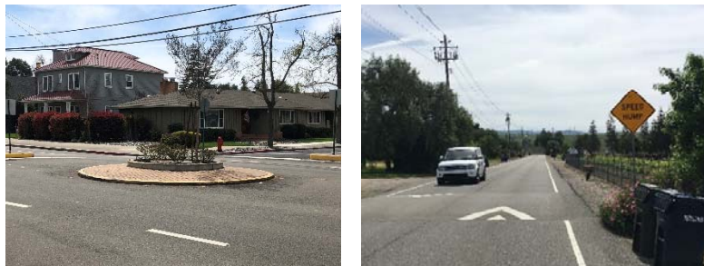
Typical bicycle boulevard features, clockwise from top left: sharrows, wayfinding, speed hump, and traffic circle
