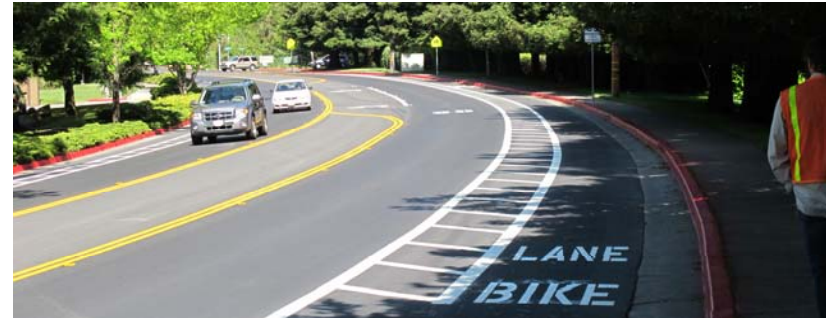
A typical buffered bicycle lane
