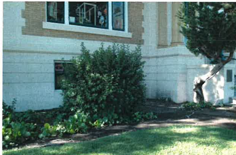
Figure 6. Above: An example of a shrub that blocks windows and obscures the building base.
