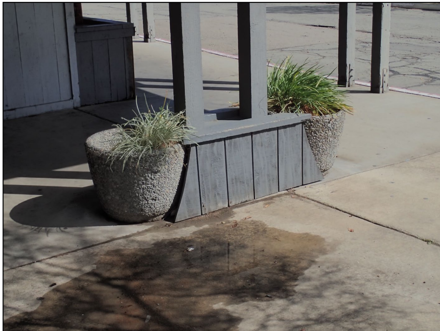
Vineyard Shopping Center. Primary building. Paired pebble-clad concrete planter with T-111 plywood accent. Representative example. View east. LSA photograph 3/18/25.
