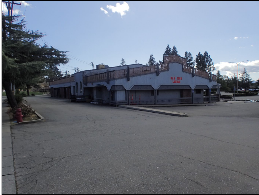
Vineyard Shopping Center. Secondary building. North and east façades. View southwest. LSA photograph 3/18/25.
