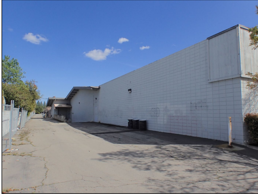
Vineyard Shopping Center. Primary building. Western anchor tenant space, north (rear) façade. View east. LSA photograph 3/18/25.
