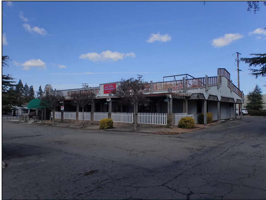
Vineyard Shopping Center. Secondary building. West and south façades. View east. LSA photograph 3/18/25.
