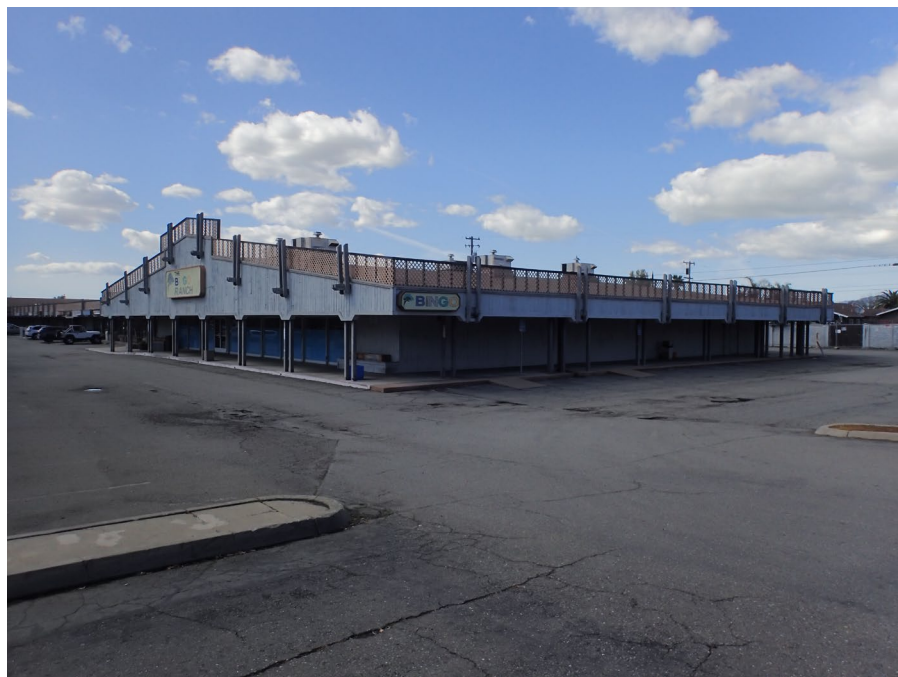
Vineyard Shopping Center. Primary building. Anchor tenant space, far right side of south façade (partial) and east façade. View west. LSA photograph 3/18/25.
