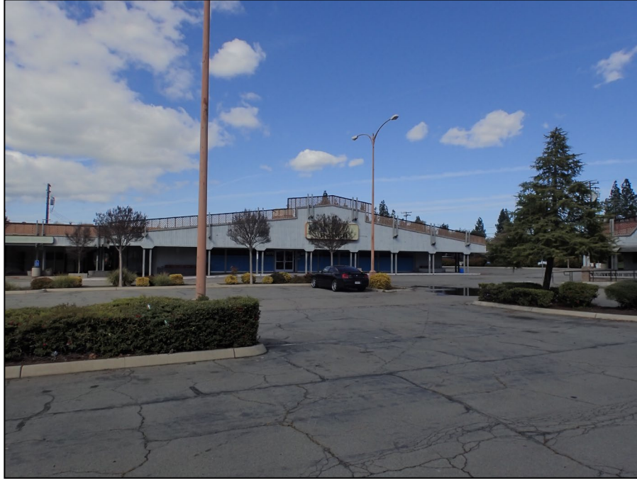
Vineyard Shopping Center. Primary building. Anchor tenant space, far right side of south façade (partial). View northeast. LSA photograph 3/18/25.
