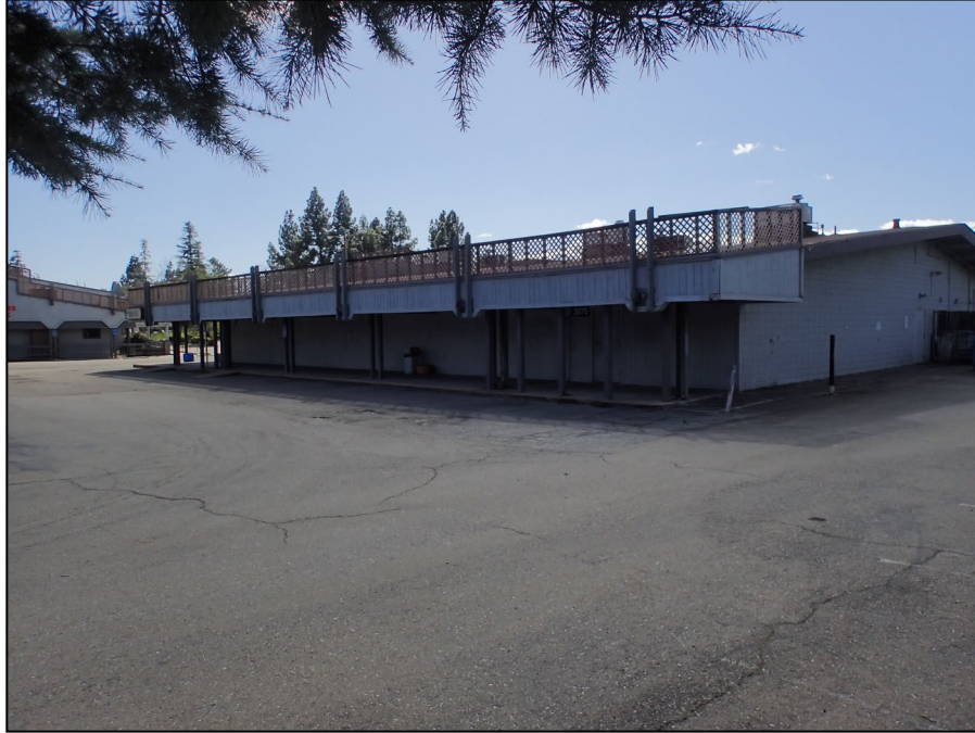
Vineyard Shopping Center. Primary building. Anchor tenant space, east façade and portion of north façade. View southwest. LSA photograph 3/18/25.
