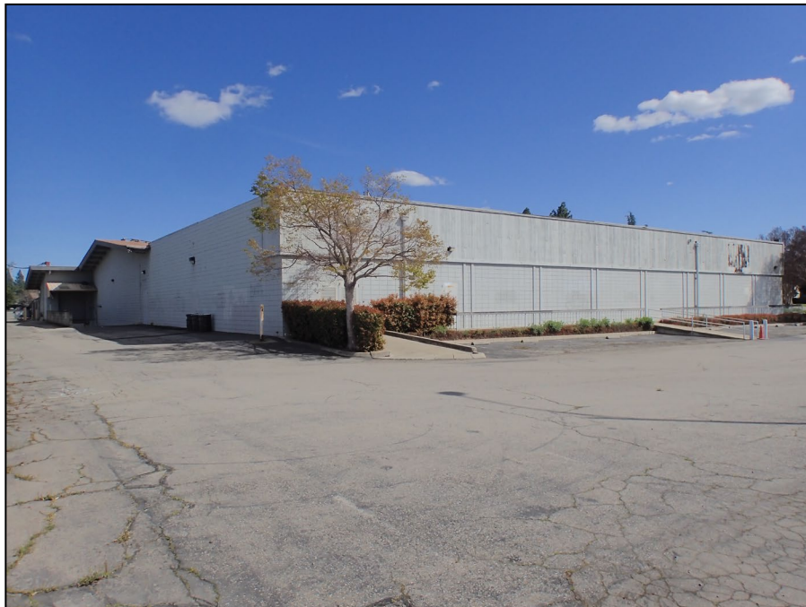
Vineyard Shopping Center. Primary building. Western anchor tenant space, northern (rear) and west façades. View southeast. LSA photograph 3/18/25.
