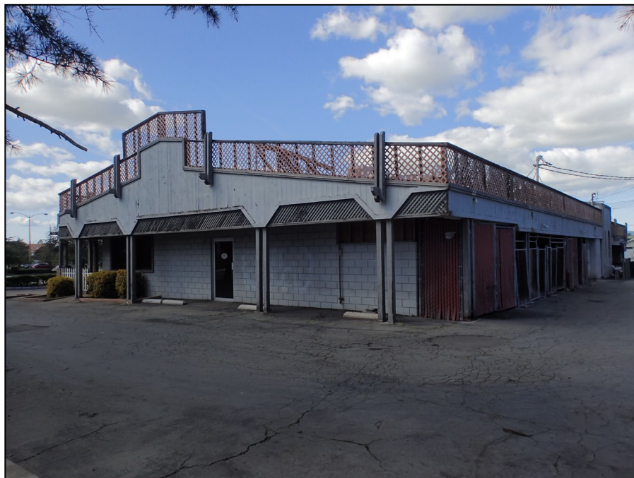
Vineyard Shopping Center. Secondary building. South and east façades. View northwest. LSA photograph 3/18/25.
