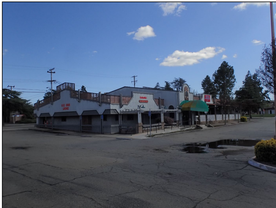
Vineyard Shopping Center. Secondary building. North and west façades. View southeast. LSA photograph 3/18/25.
