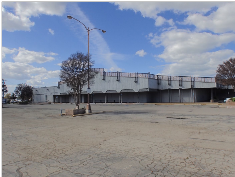
Vineyard Shopping Center. Anchor tenant space, far left side of south facing façade. View northwest. LSA photograph 3/18/25.
